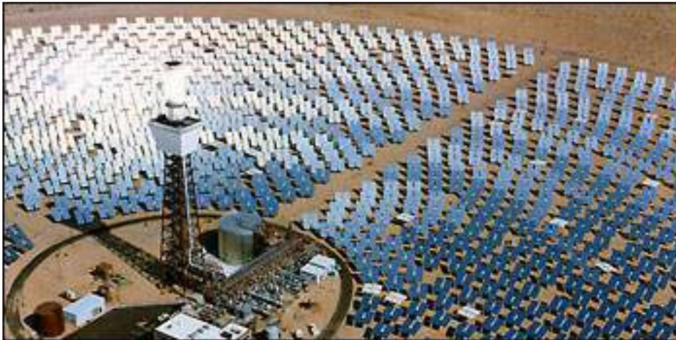
Solar one (1982-88) → Two (1996-99): 10 MW power capacity
